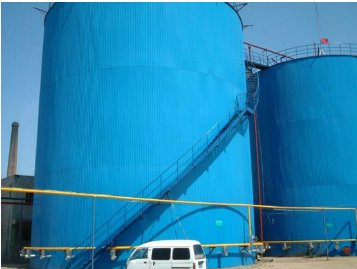
Rizhao. The biogas tank utilizing the waste water of the liquor production
